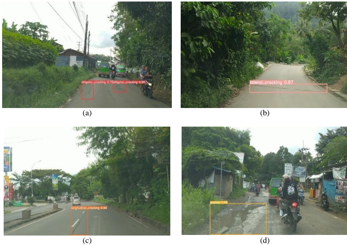
Figure 5. Example of road damage detection results using the YOLOv9-based model for multiple damage classes: (a) alligator cracking class, (b) lateral cracking class, (c) longitudinal cracking class, (d) pathole cracking class
